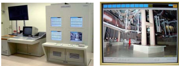
Fig. 9 Synthetic Sodium Leak Monitoring System
