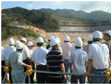
【Site Tour: Tsuruga NPP No. 3 & 4 units (under construction)】
